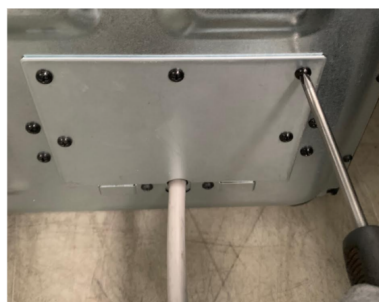
Assemble cover and tighten screws.
